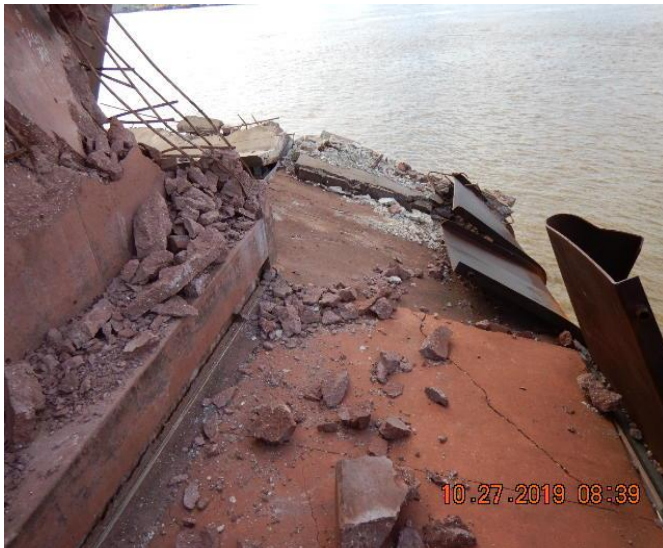
Picture 7 – Before Demolition
