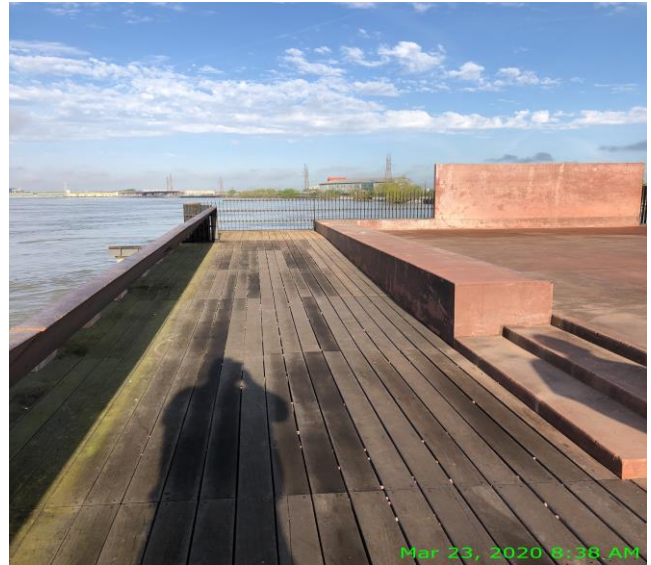
Picture 6 – After Demolition and Clean-up
