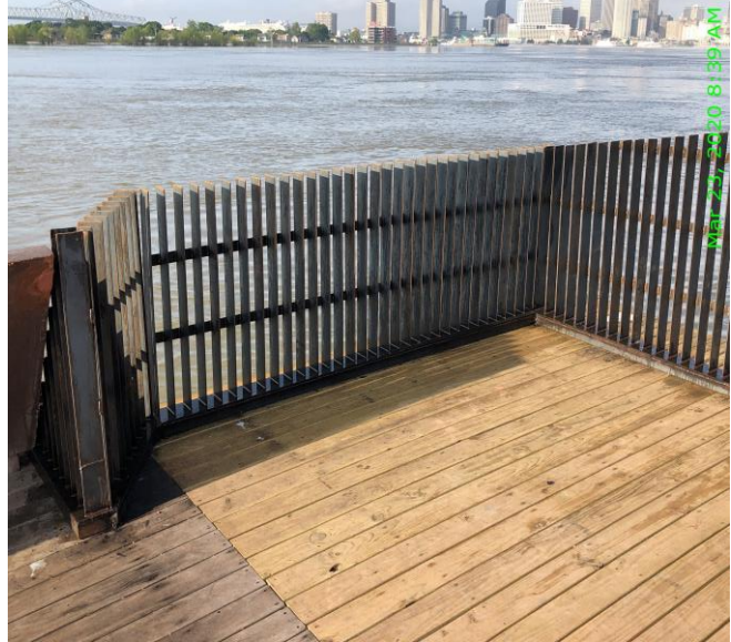
Picture 2 – After Demolition and Clean-up
