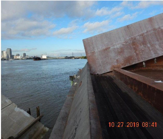
Picture 5 – Before Demolition
