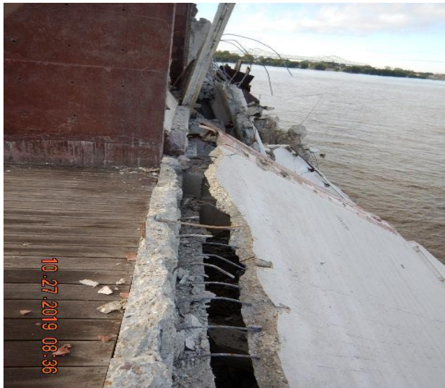
Picture 3 – Before Demolition
