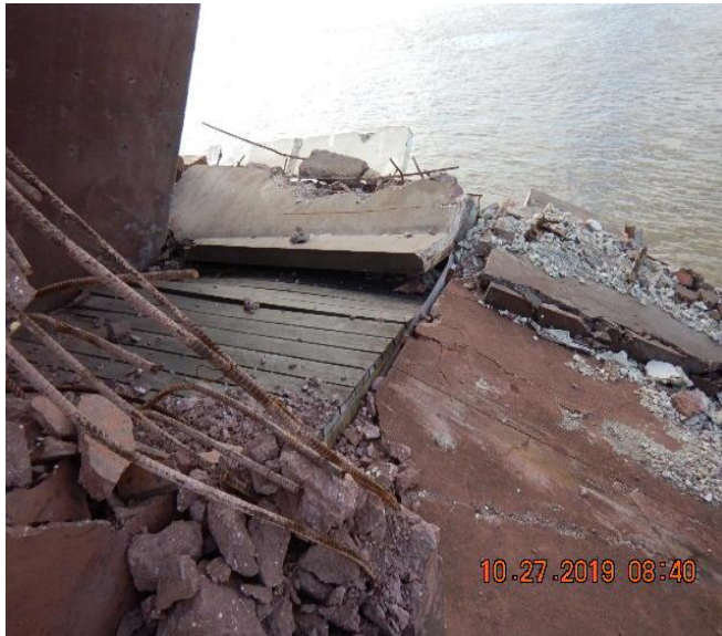
Picture 1 – Before Demolition
