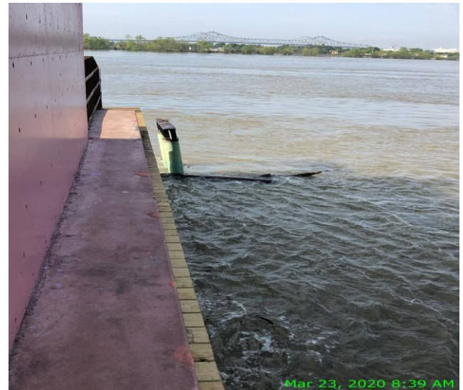
Picture 8 – After Demolition and Clean-up
