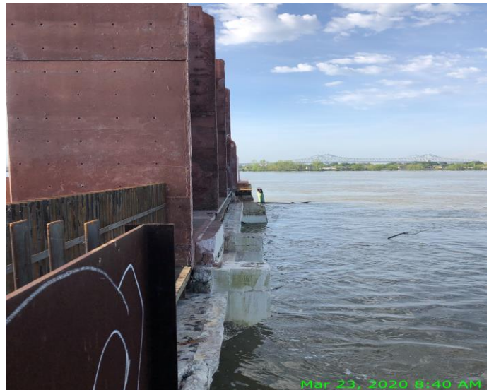
Picture 4 – After Demolition and Clean-up
